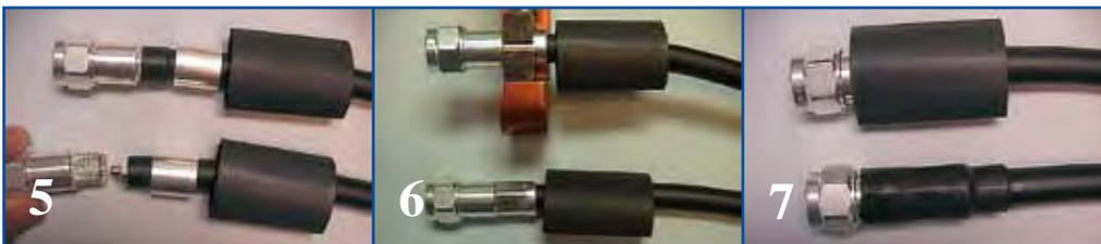
**Step 5:** Slide the connector over the end of the core and push it up to the end of the jacket. Rotate the connection back and forth in a clockwise-counter clockwise motion in reference to the axis of the cable until the back of the connector works its way under the end of the jacket. Now push the connector onto the cable with some back and forth motion until it stops.
